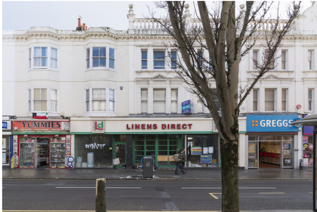
Photo of Western Road retail unit frontage taken before the works
